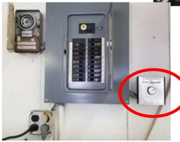
The Manager will turn on the vent hood over the grills - The fan is controlled by a variable speed switch located to the right of the main power panel (back wall behind the steam table).
